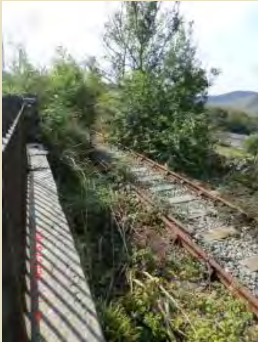
Left: Just south of Blaenau. At grade / low embankment. A bit of ground clearance and we could have a 57xx running here tomorrow! If only it was that simple...
