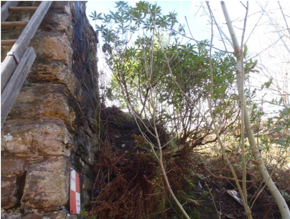
Photo 21 typical bush/sapling at wingwall quoins 11/02/2014
