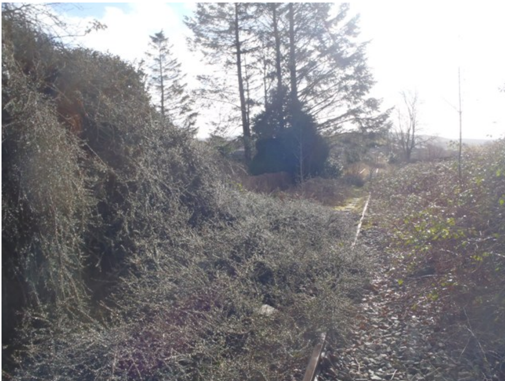
Photo 20 track view looking towards Trawsfynydd 11/02/2014
