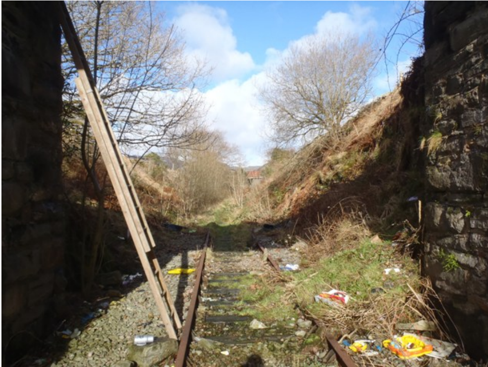
Photo 19 track view looking towards Blaenau 11/02/2014
