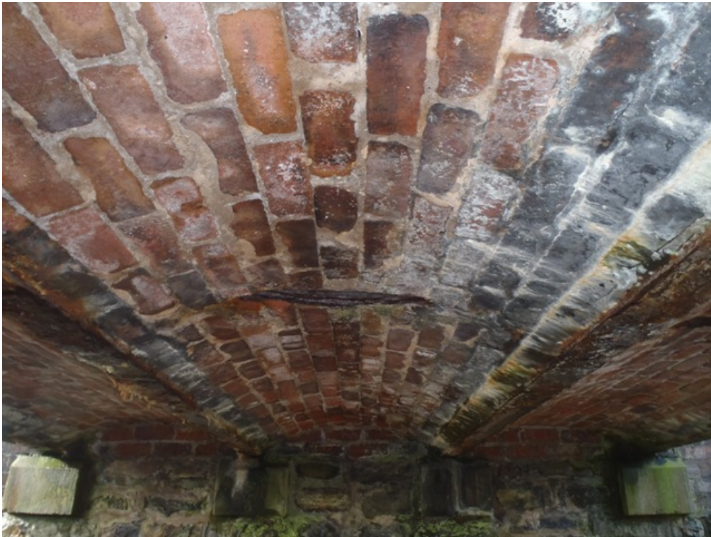
Photo 5 general view of soffit 11/02/2014
