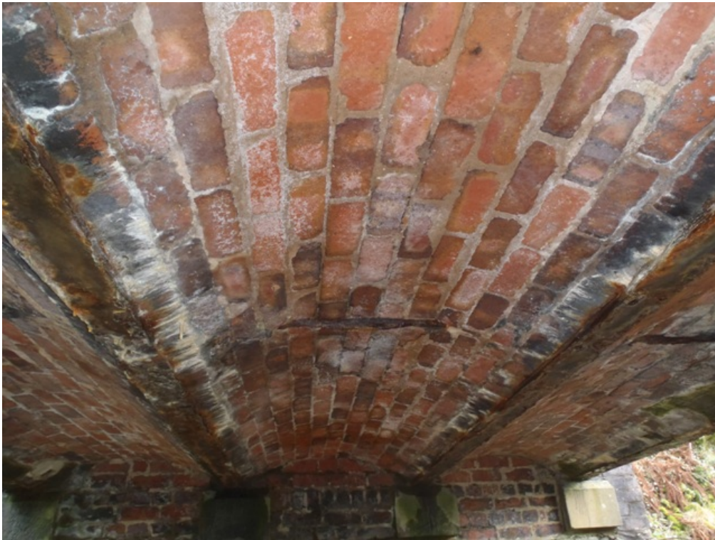
Photo 5 general view of soffit 13/02/2014
