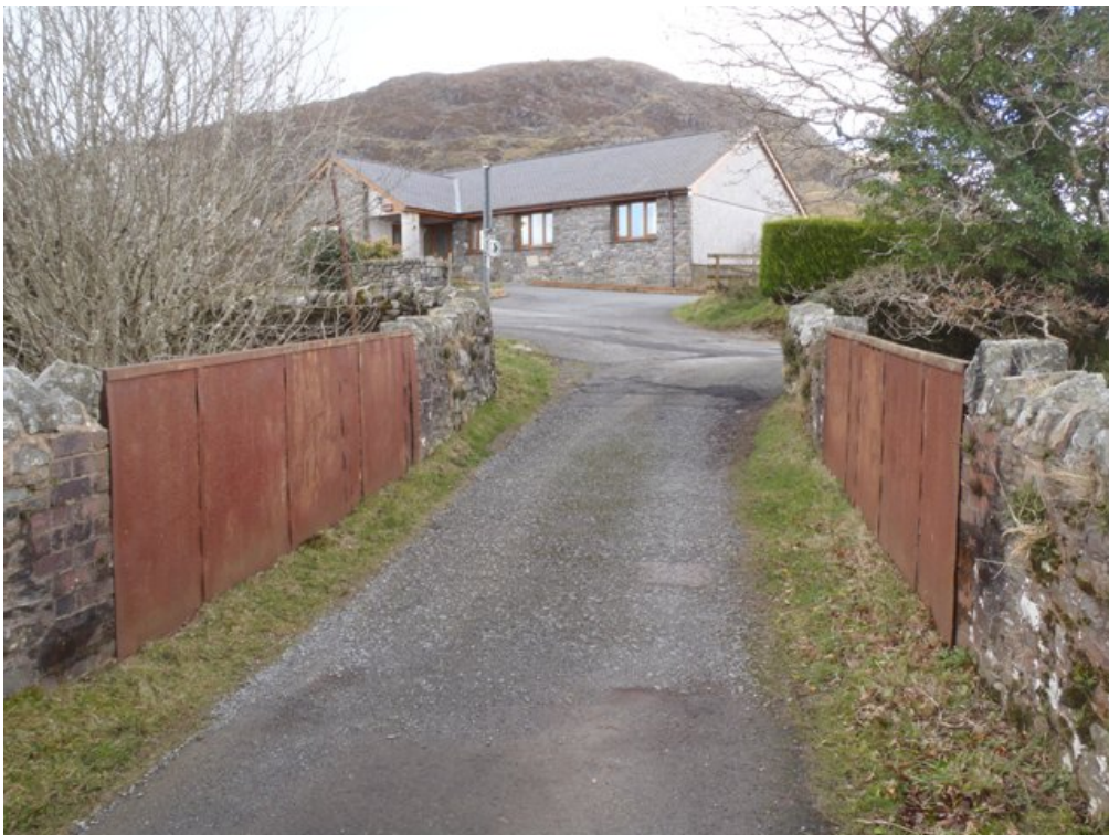
Photo 4 road over looking towards downside 13/02/2014
