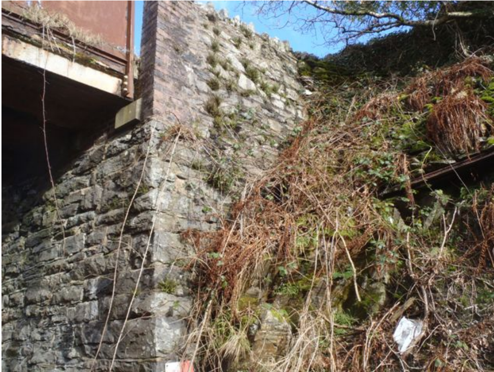
Photo 23 vegetation at wing walls 13/02/2014
